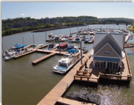
2 Story, Marina Offices, Restrooms, & Vending
