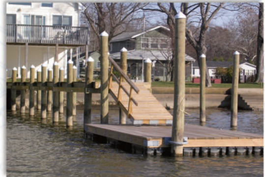
Pier and Wood Ramp in Maryland
